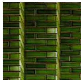
Dark green glazed Brickwork
