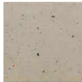
4. Precast concrete horizontal bands
