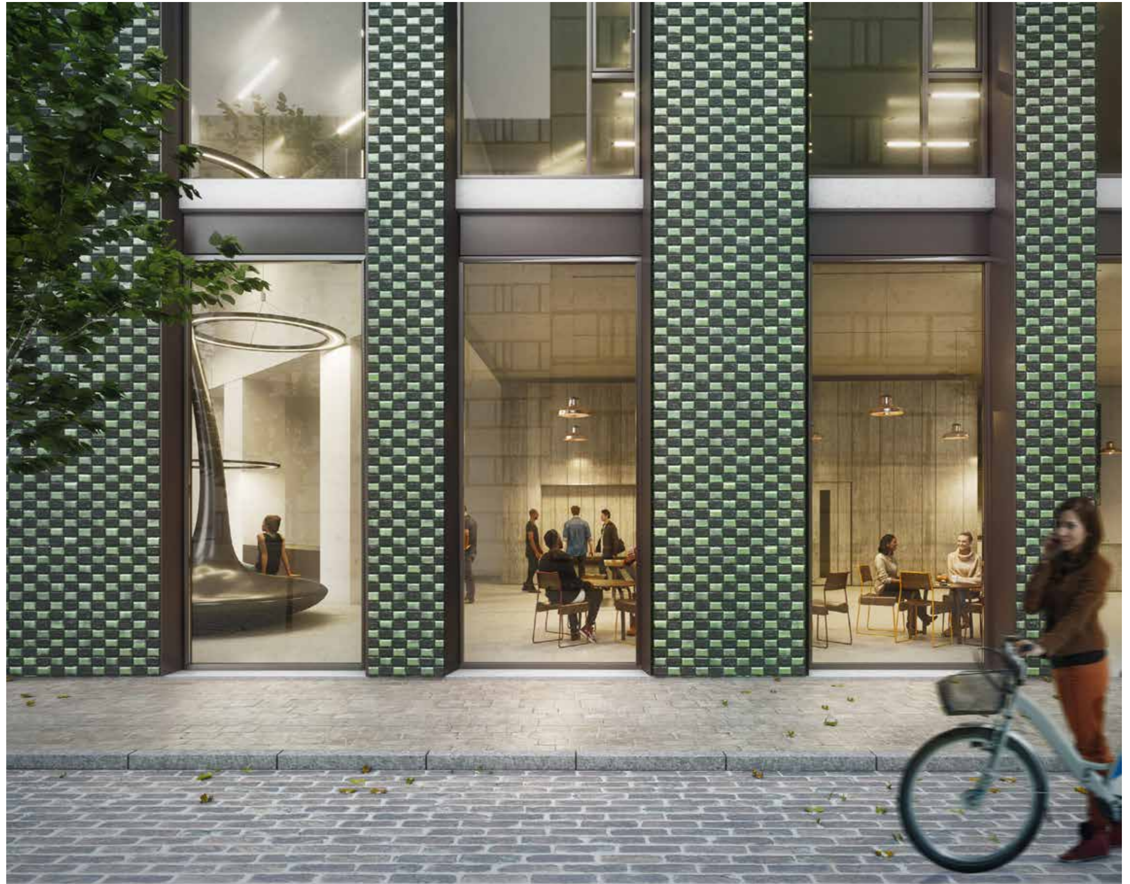
Detail View of the black and green glazed headers bond at ground floor
